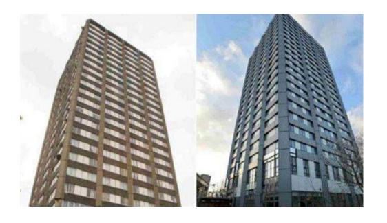
Between 2014 and 2016 the façade was renovated applying a ventilated cladding system with PU as insulation boards. The airgap was equipped with fire barriers and windows also replaced.
