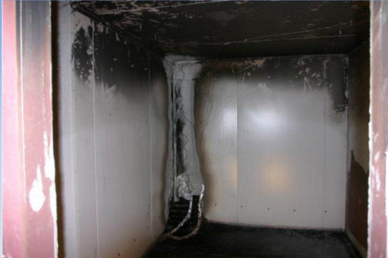
Figure 9. Damage to corner specimens with skins and bolting in place.
